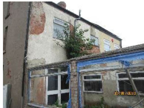
Rear elevation – some elements to be demolished
